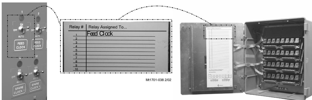
**Figure 110. Relay Assignments**
